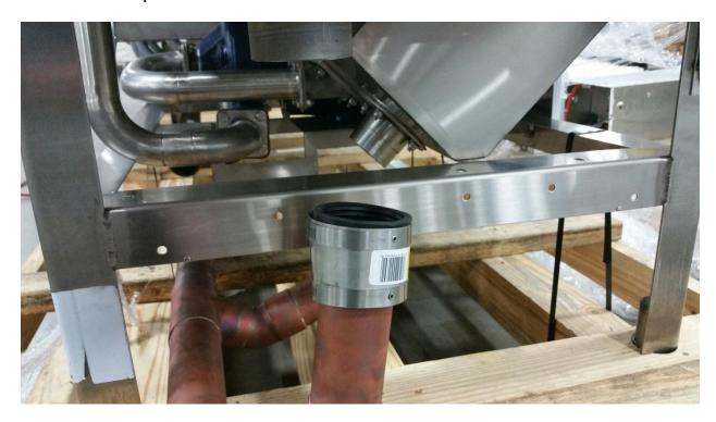
Use a cardboard box or packing materials placed under the manifold to hold it in place. Once all the connection points are lined up and the no-hubs are all centered on the joint, tighten each by turning the screws on top and on bottom evenly. Avoid tightening one all the way, then trying to tighten the other. The hub will bind and be uneven.
