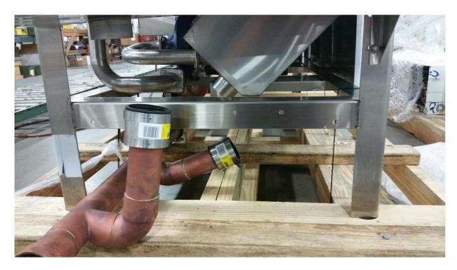
Place the manifold on the machine after removing the machine from the pallet. Attach the "J" hooks to hold the manifold in place before attaching building drains. Avoid "U" turn bends or tight elbows.
